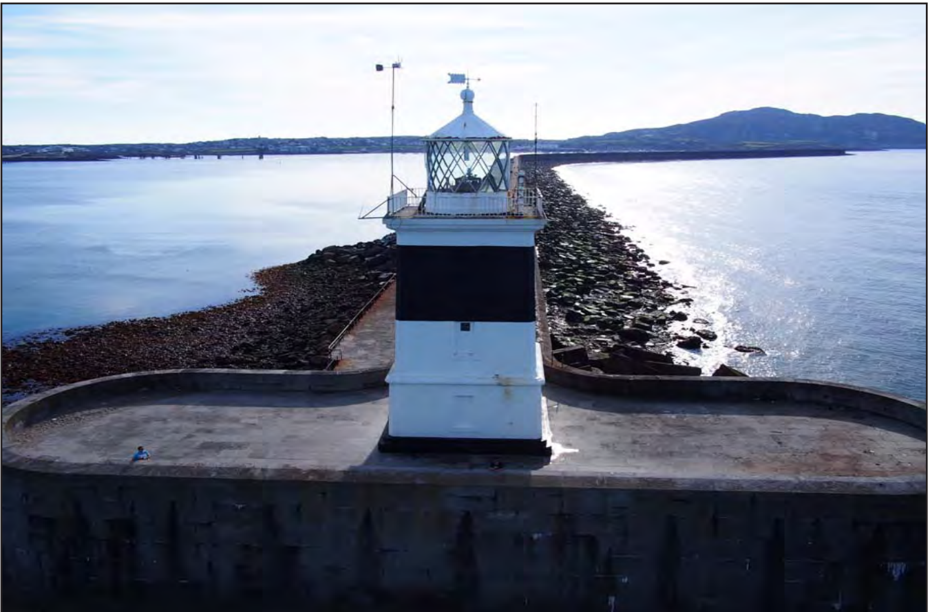
Plate 14: View of full length of breakwater showing its curve leading towards landsend at Holyhead Mountain (sourced from Civil Engineering Solutions: 20150928 Holyhead Breakwater 160.jpg).
