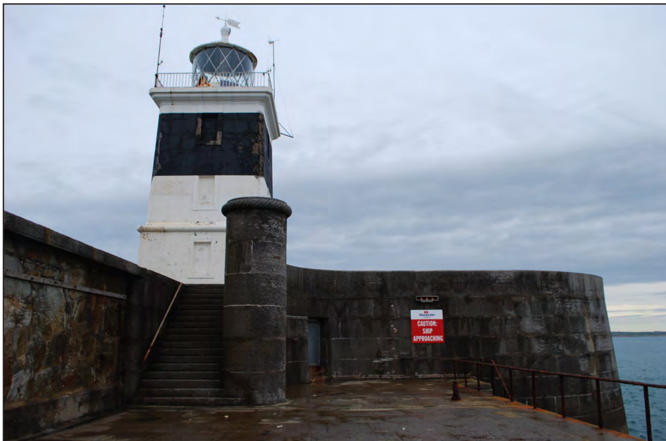
Plate 25: Holyhead Breakwater - view from west of the lighthouse (archive image: G2498_025)
