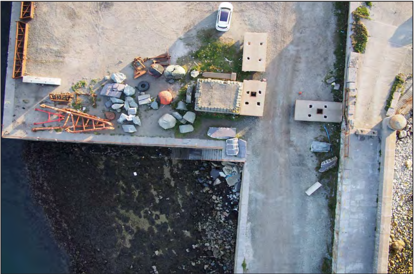
Plate 01: Holyhead Breakwater's Landsend with view of the remnants storage and working area on the portside and decorated bollard on the seaward (sourced from Civil Engineering Solutions: 20150928 Holyhead Breakwater 988.jpg).
