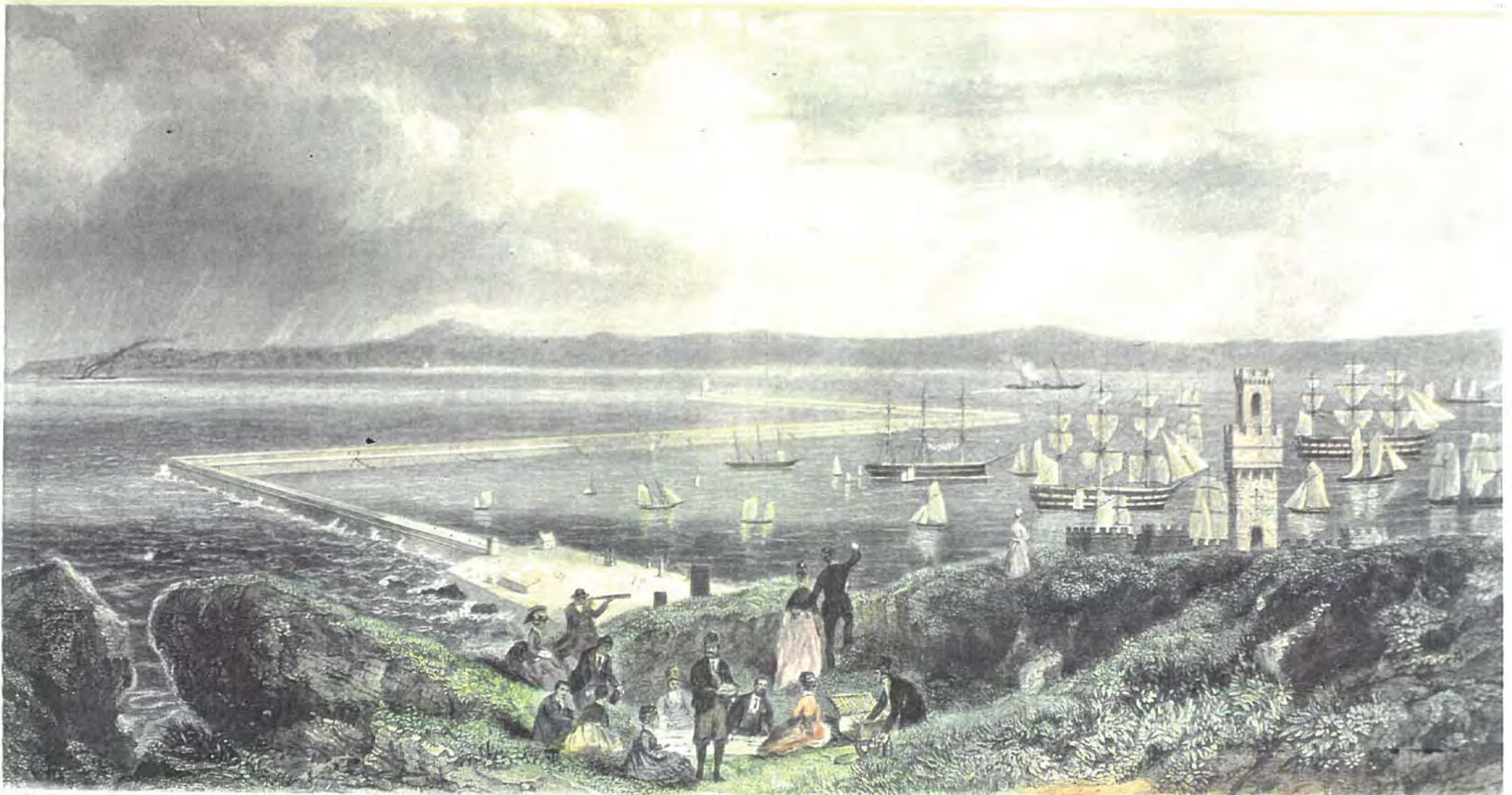
Figure 06: View of the Great Breakwater at Holyhead in 1874 shortly after its completion. Image by G.H. Andrews (NLW)
