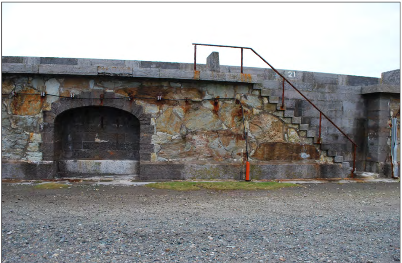
Plate 22: Holyhead Breakwater - view from south of refuge within the breakwater parapet and stairway between upper and lower levels (archive image: G2498_015).
