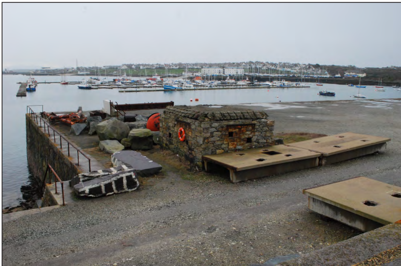
Plate 29: Holyhead Breakwater - view from north of former wharf at southwestern end of the breakwater (archive image: G2498_050).
