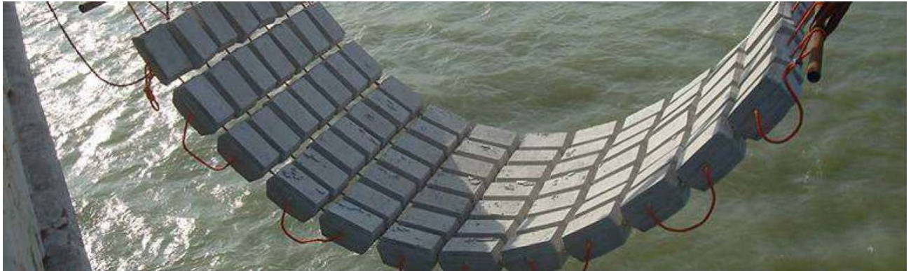
Figure 6: Example of an articulated concrete block mattress (ACBM), (Credit: Maccaferri)
