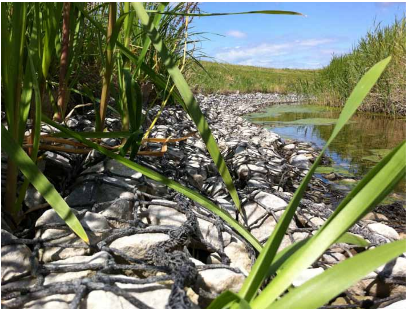
Rock Mattresses on spillway toe
