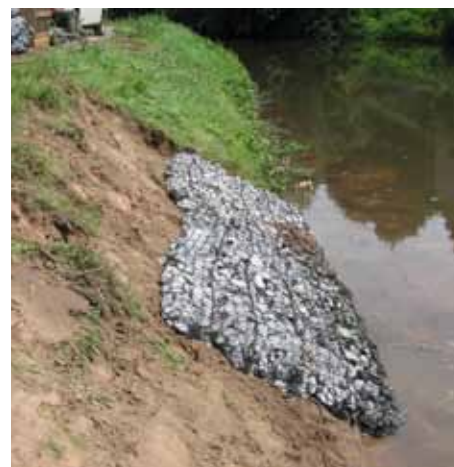
Rock Mattress placed on river bank
