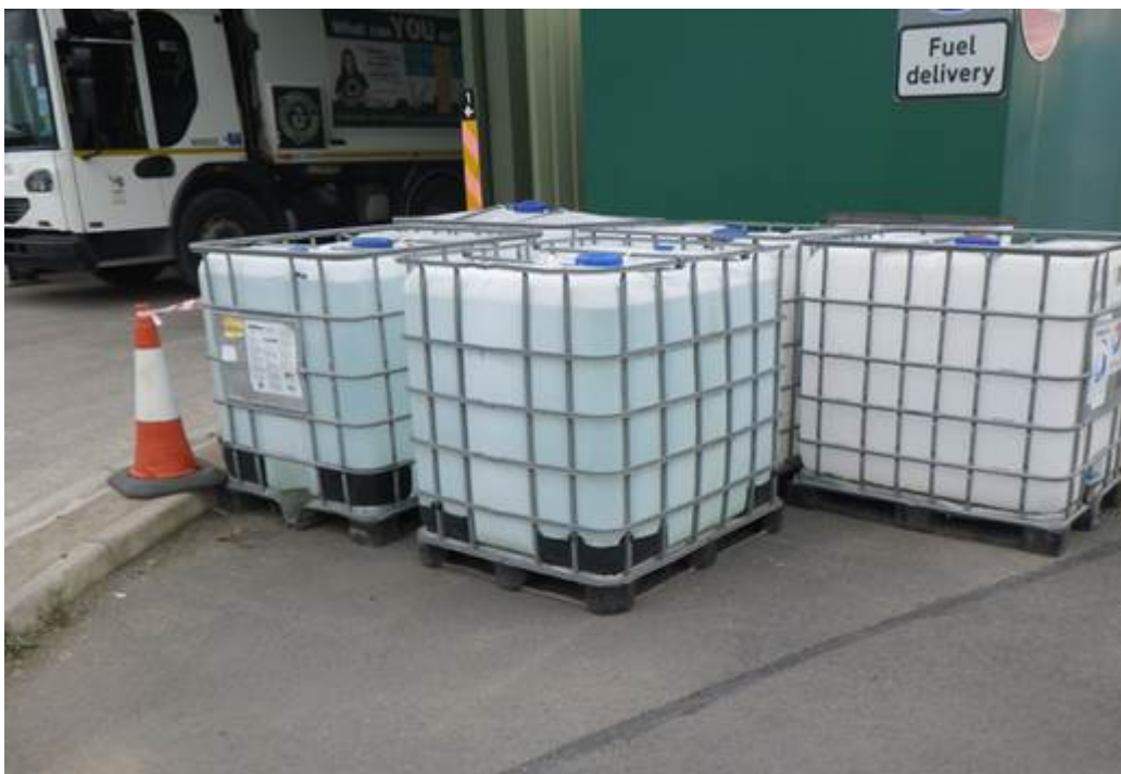
Photo 1: IBCs stored without suitable secondary bunding
