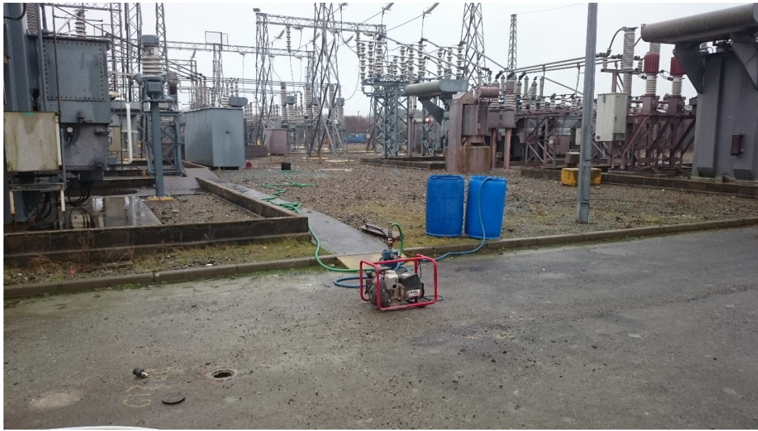
Figure 1 - Rectifier Yard Area of frozen core collection. Photograph taken during pumping operations.
