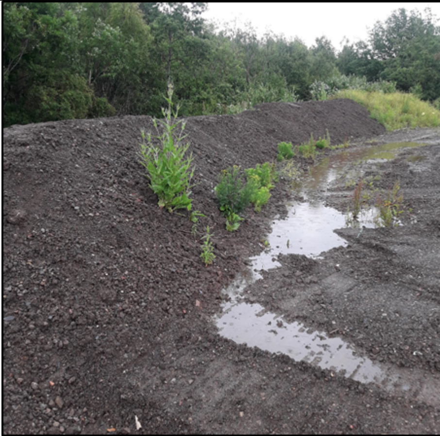
Image 3 – showing processed material deposited for use as a bund
