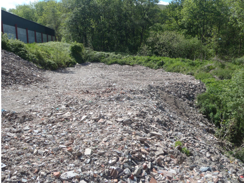
Extension to lower yard behind the new building
