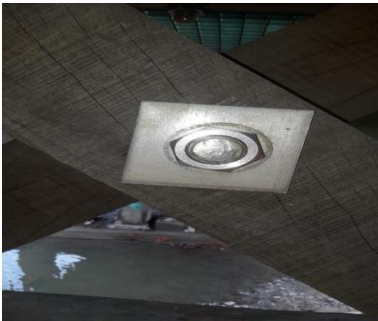
New diagonal restraint timber photo with centre bolting installed at Artro.
