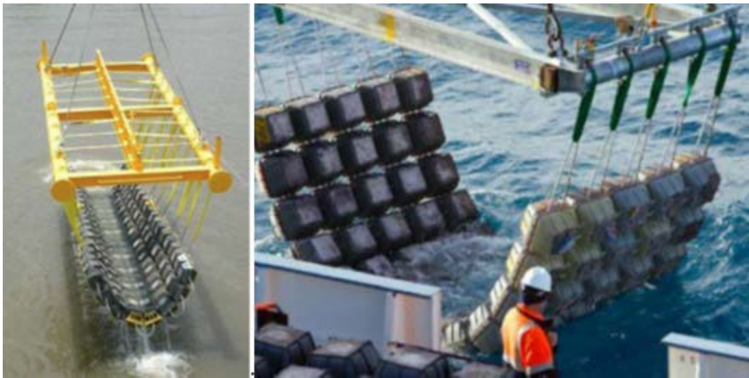
Figure 2-4 Concrete mattress deployment (courtesy of FoundOcean)
