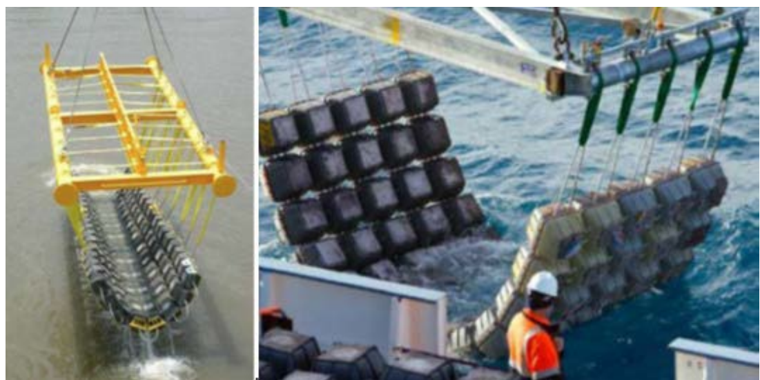
Figure 2-4 Concrete mattress deployment (courtesy of FoundOcean)
