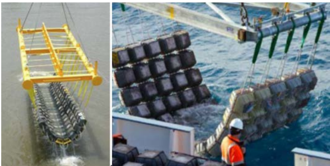
Figure 2-4 Concrete mattress deployment (courtesy of FoundOcean)
