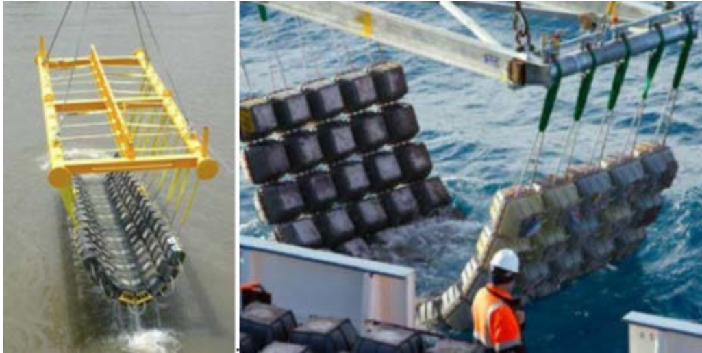
Figure 2-4 Concrete mattress deployment (courtesy of FoundOcean)
