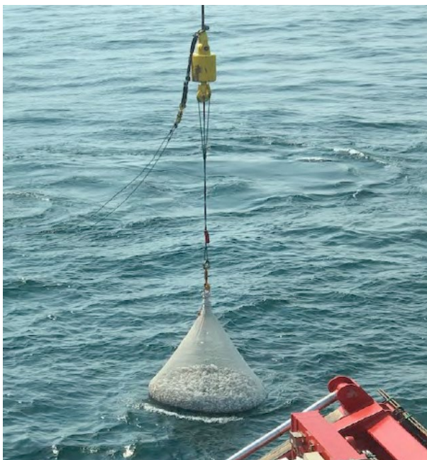
Figure 2-5 Rock bag deployment (NKT)
