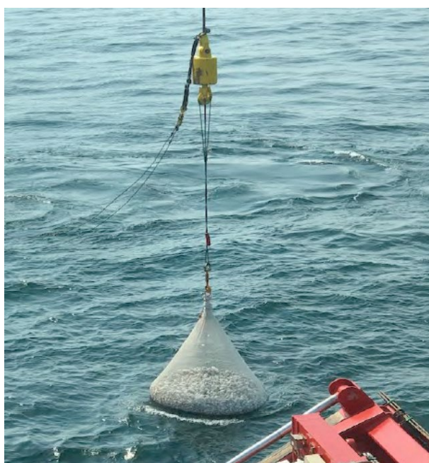
Figure 2-5 Rock bag deployment (NKT)
