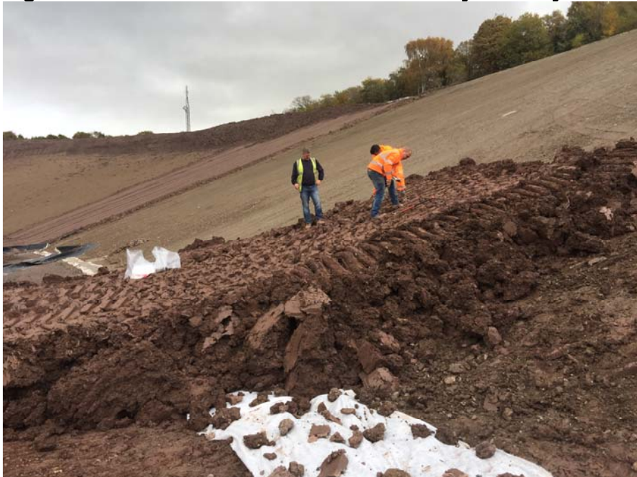
Figure 9: Side wall seal construction at Parrys Quarry Landfill site
