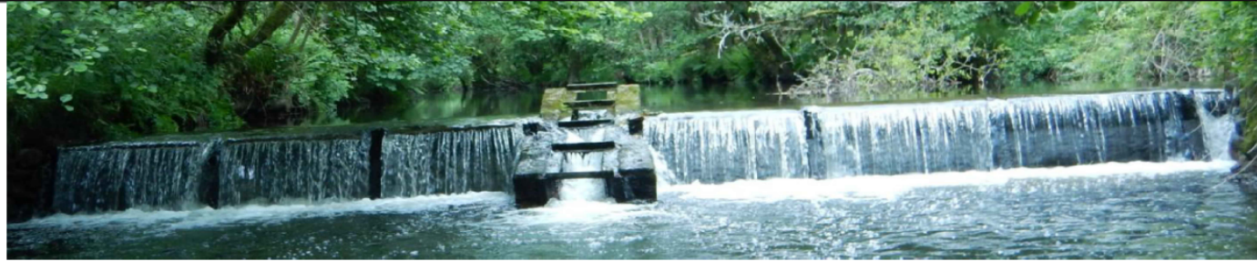
VIEW OF WEIR LOOKING UPSTREAM
