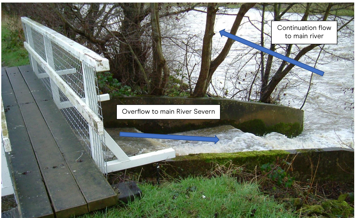
Photo 6: Overflow from open channel back to main River Severn
