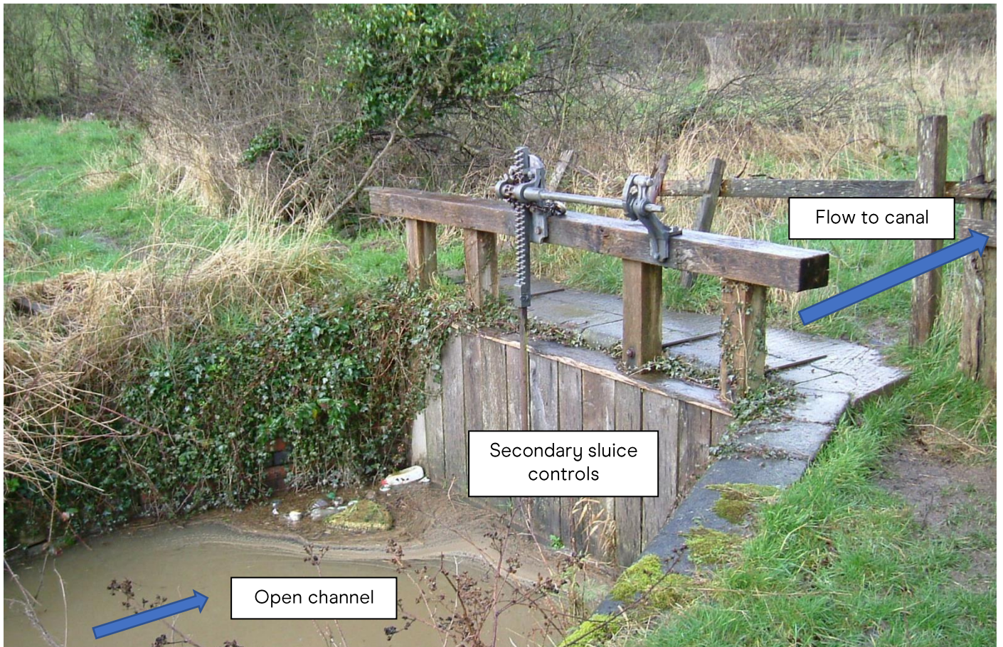
Photo 7: Secondary sluice controls to canal
