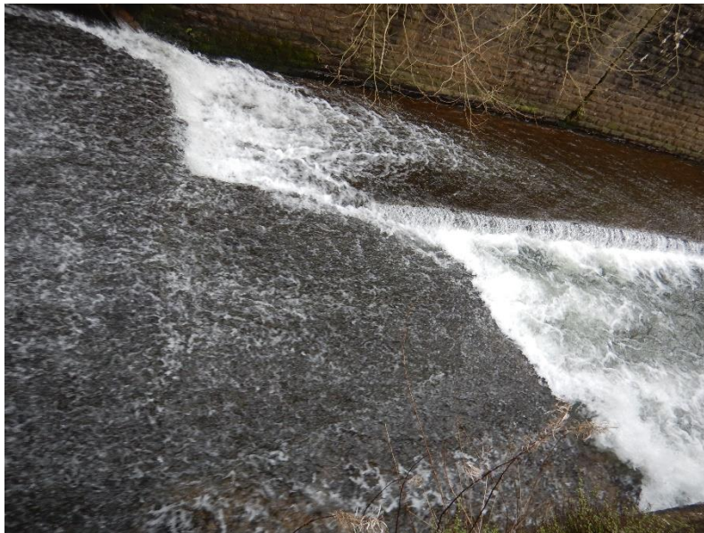
Figure 2: Lower part of the weir including concrete plinth running along the left-hand bank
