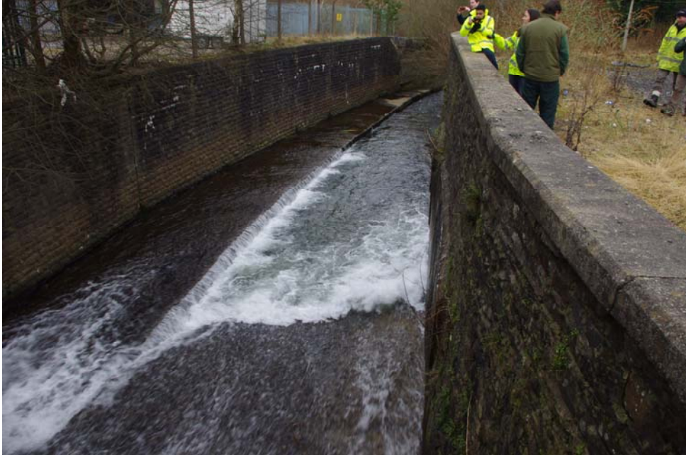
Plate 2.2 Apron downstream of Gas Works weir
