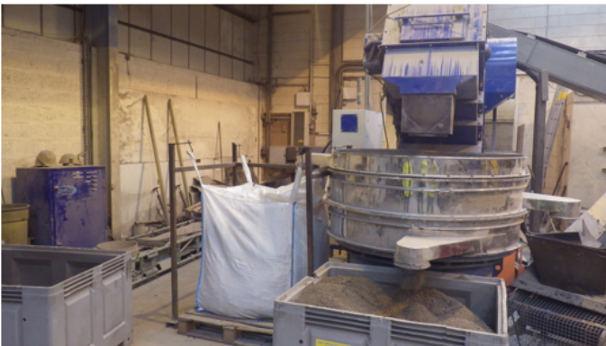
Photograph 6. Line 4 located further away from the wall.
