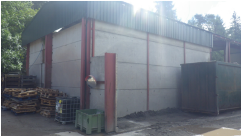
Photograph 1 Large stockpile of fines removed from side of CRT building
