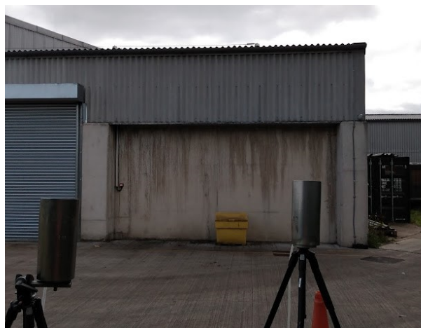
Downwind location 2 – Position of the downwind sampler, looking towards MBT facility Biofilters
