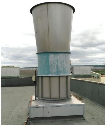
Figure 3-3 – Example axial extract fan
