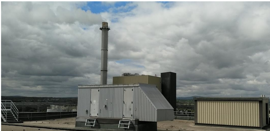
Figure 3-8 – Boiler 7 chimney as viewed from RCF3 roof
