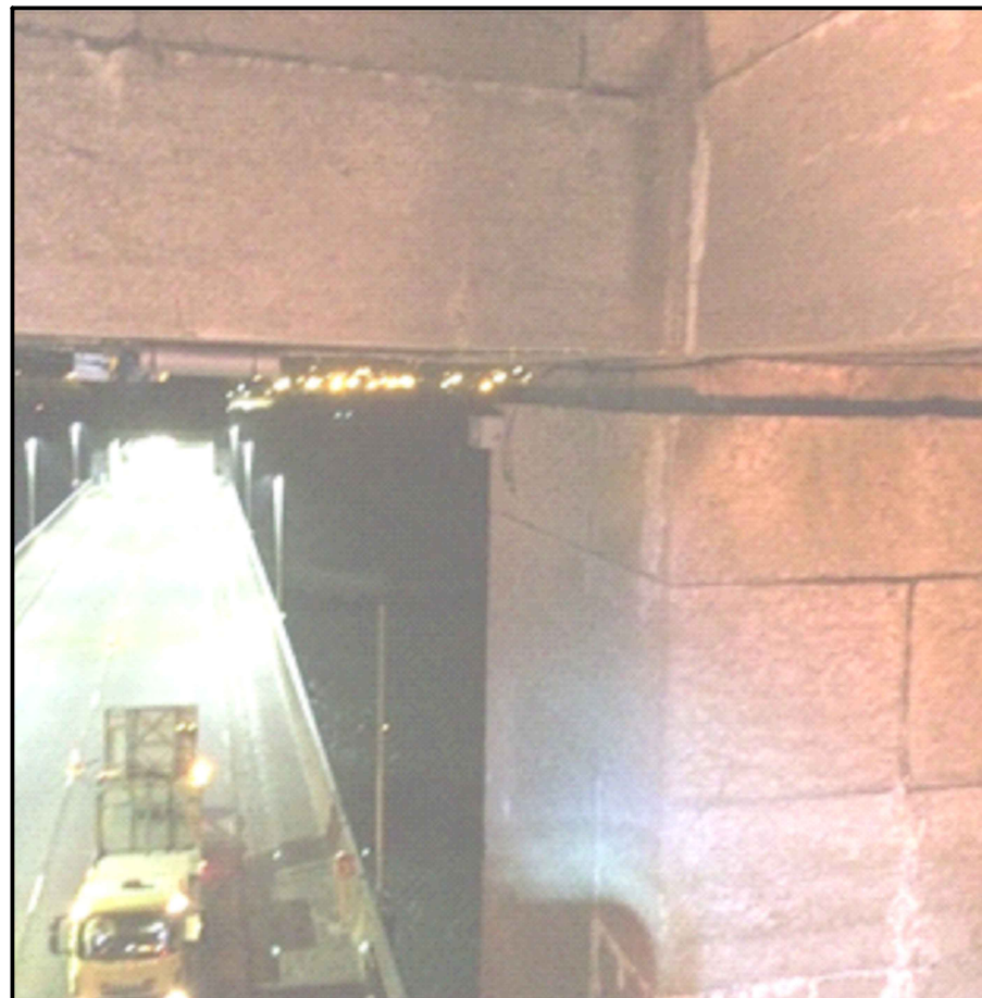
PHOTO 2 - CAERNARFON TOWER, VIEW ON TO CARRIAGE WAY
