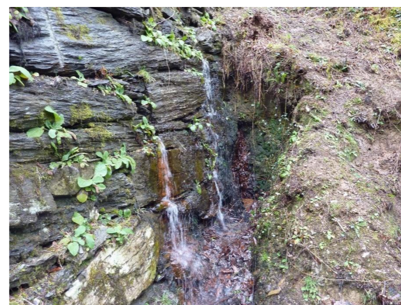
e) Leakage through the northern end of the dam
