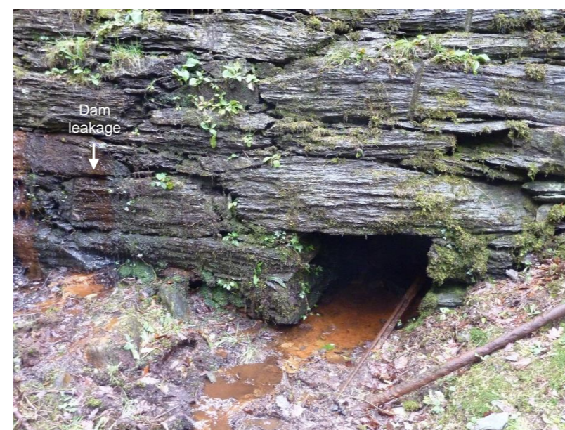
c) Low level outlet, associated with possible former drawdown facility
