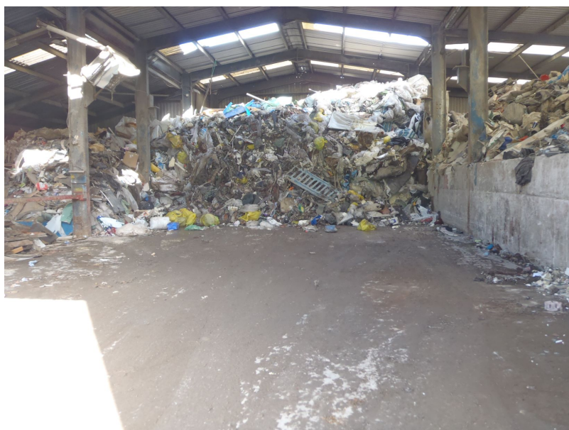
View of waste acceptance bay
