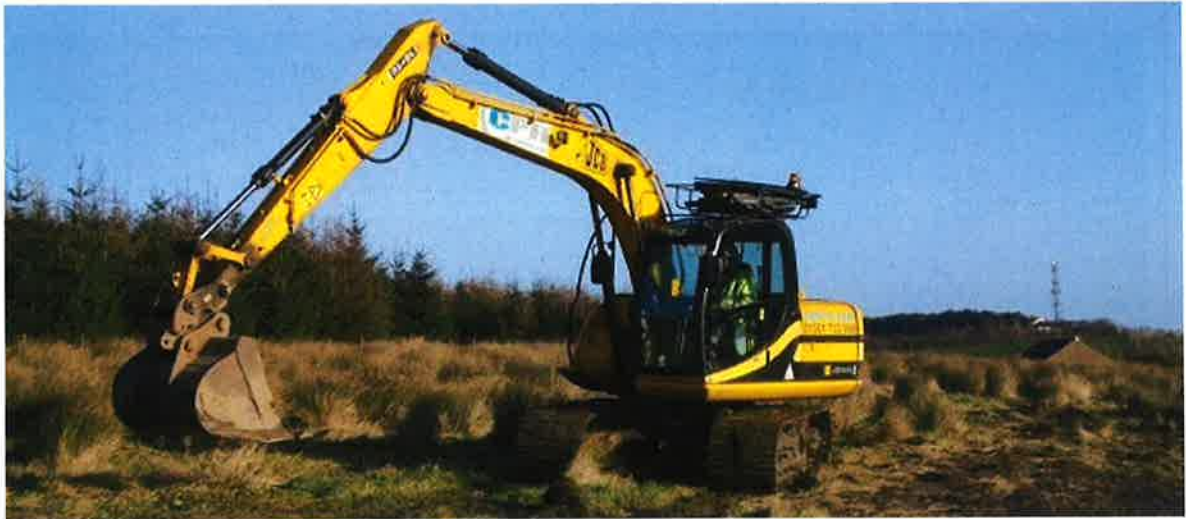
Figure 3 – Tracked 360 degree excavator
