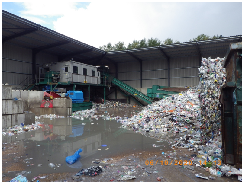
Photo of the new building on-site to enable new lines to be accepted.
