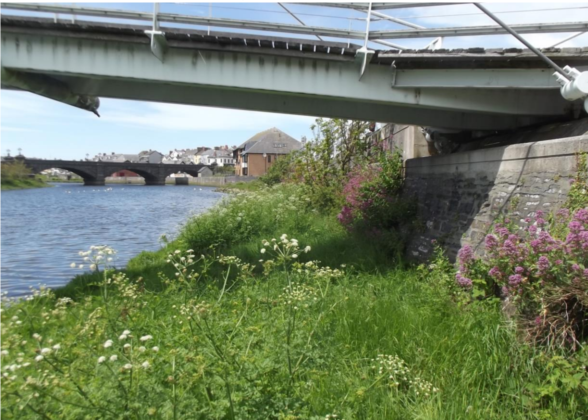
River bank at northern end of bridge
