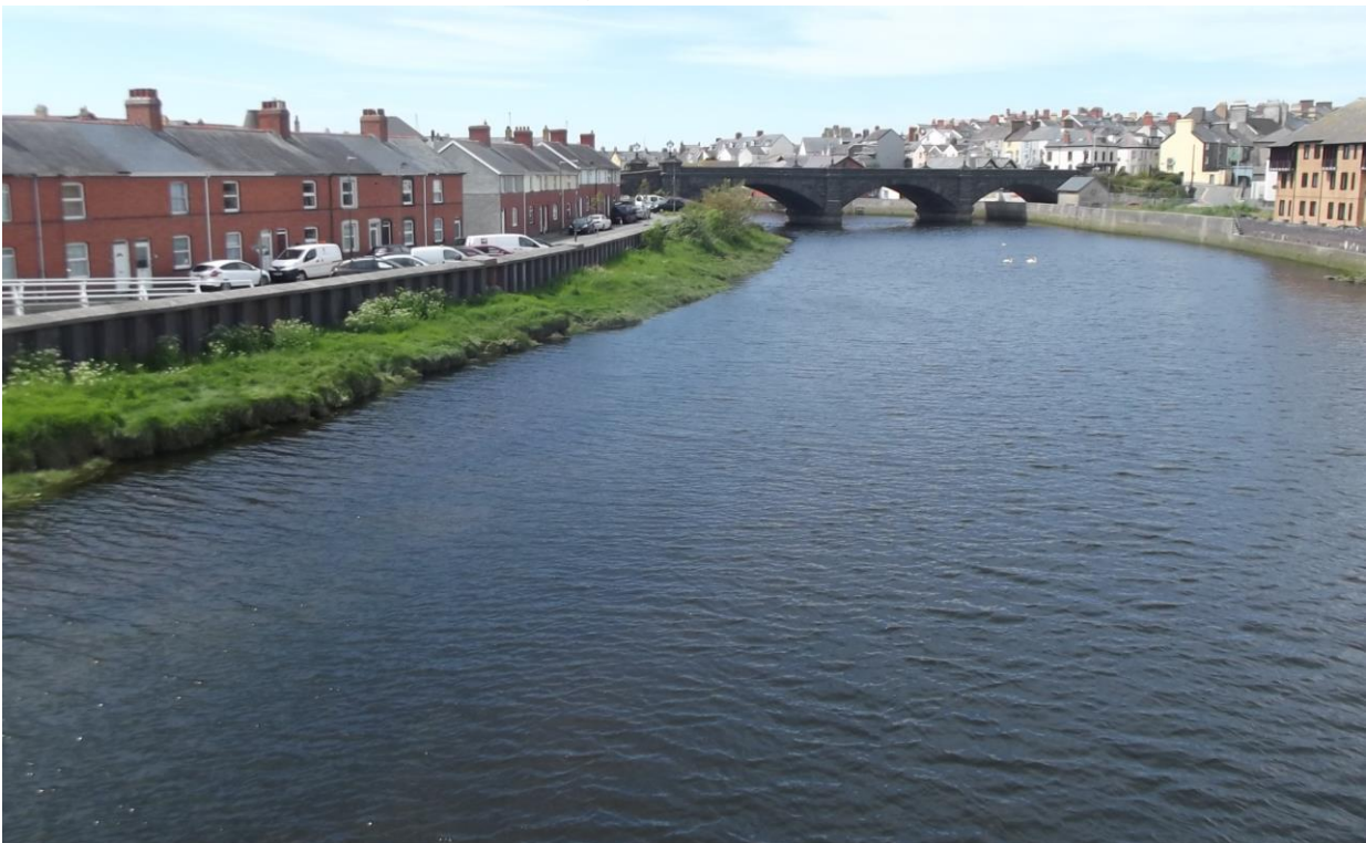
Downstream view from centre of bridge
