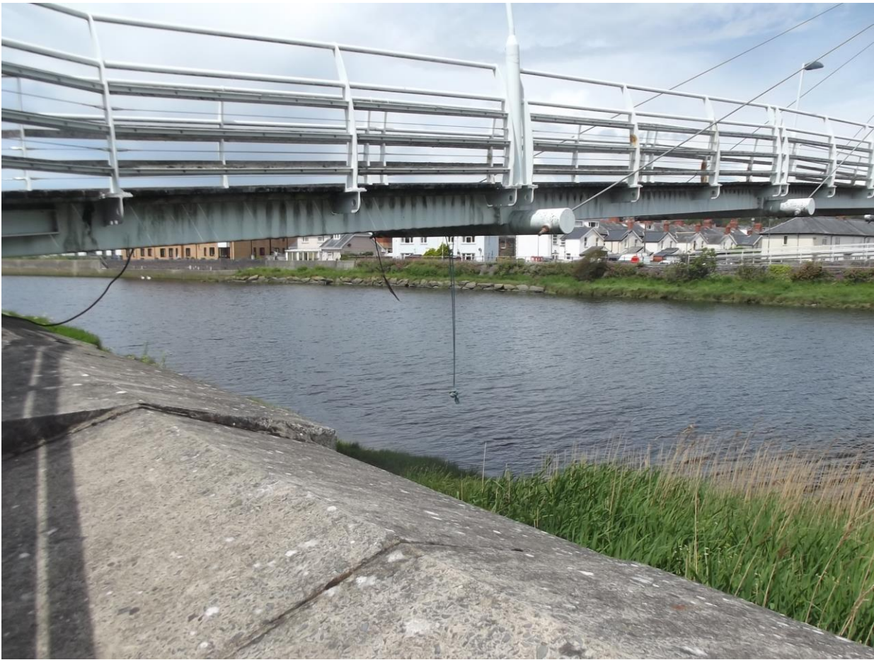
River bank at southern end of bridge
