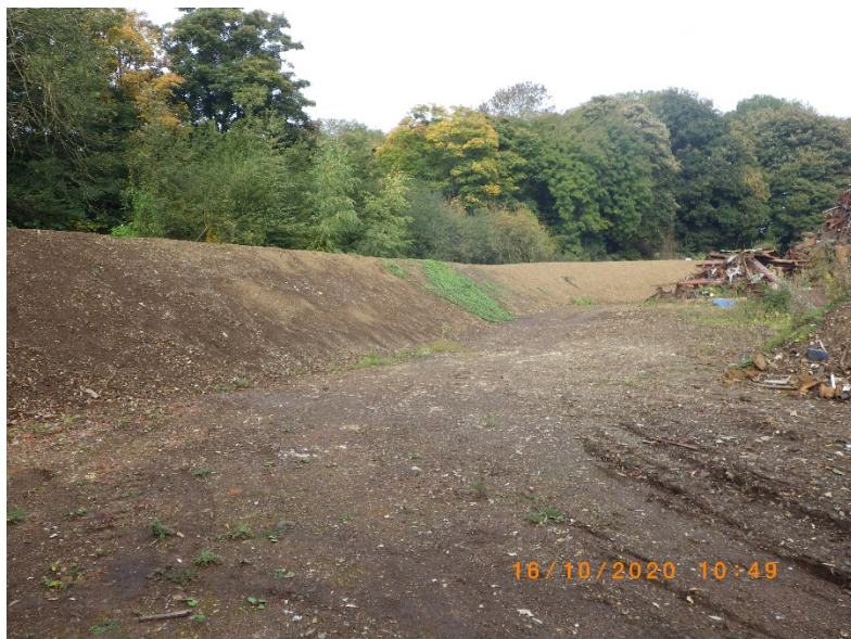
Bund at the rear of the yard
