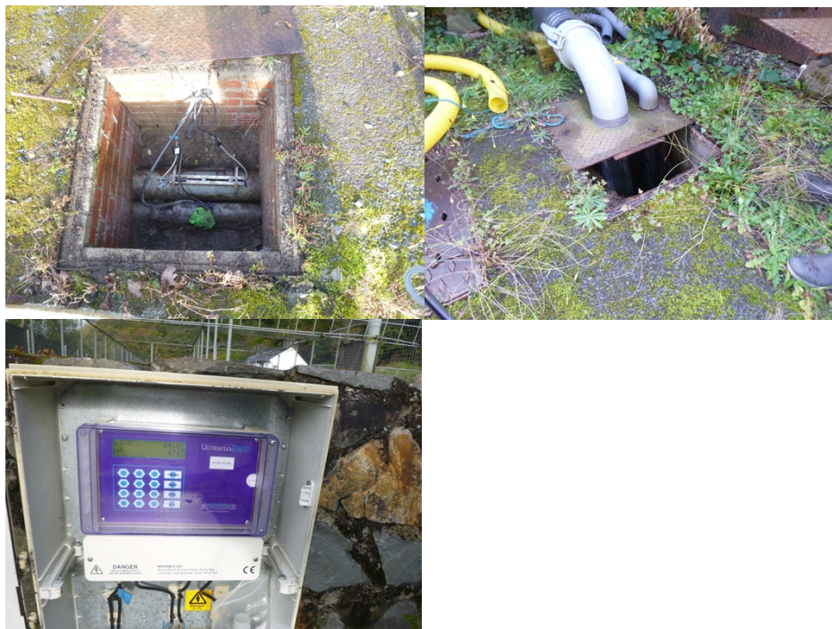
Figures 1, 2 & 3: Inspection of meters and inspection chamber.
