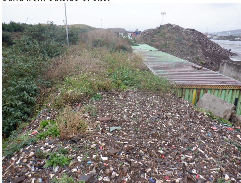
view of southern perimeter waste bund from outside of site.
