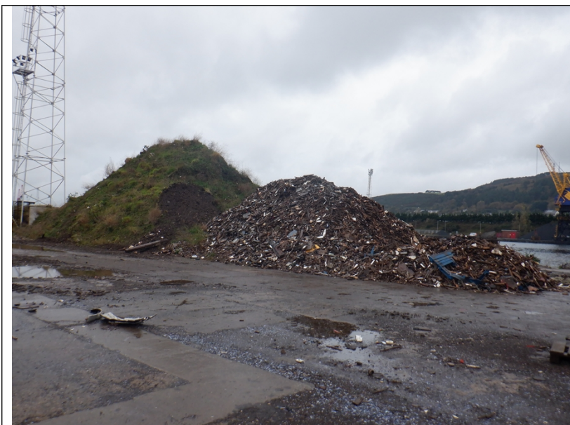
Rear of site looking north west.
