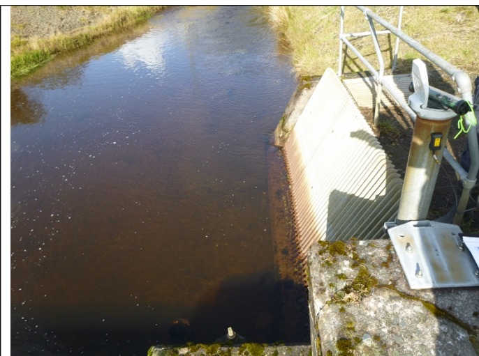
Figures 9 & 10: Orifice Plate and Abstraction Screen at Afon Llywernog
