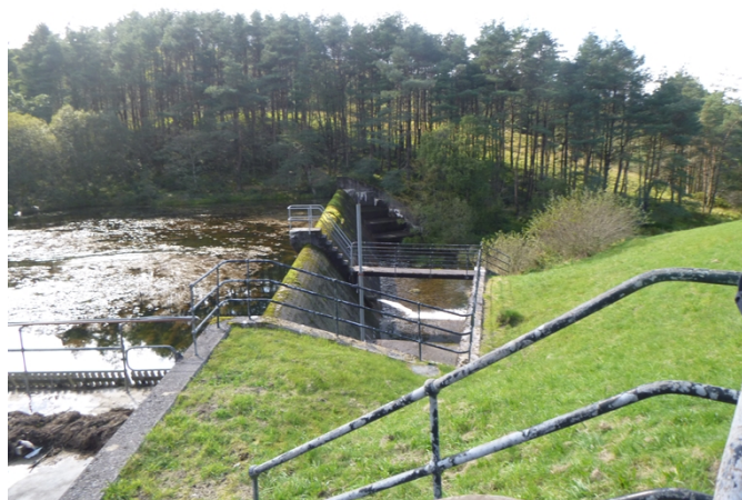
Figures 5 & 6: Afon Castell Intake and Weir
