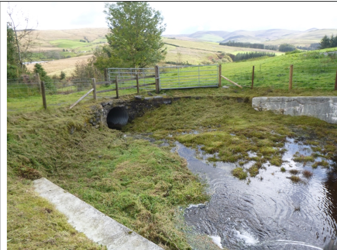
Figures 7 & 8: Orifice plate and downstream flow at Nant y Bog
