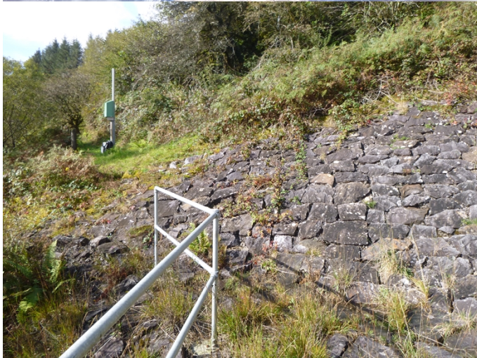
Figures 1 & 2: Staff Gauge and Access to Viewing Platform
