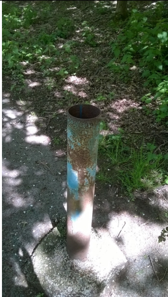
Unlabelled borehole with missing cover and lock.
