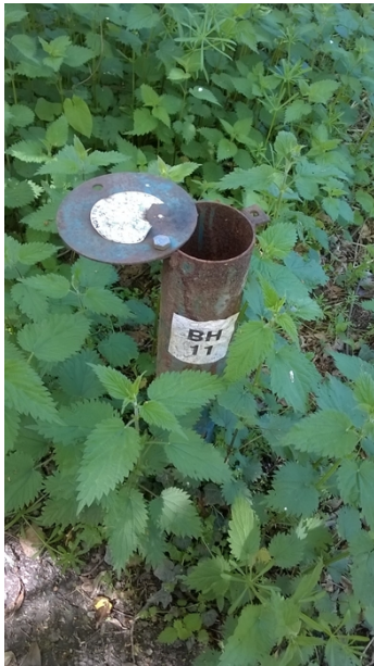
Borehole with missing lock.
