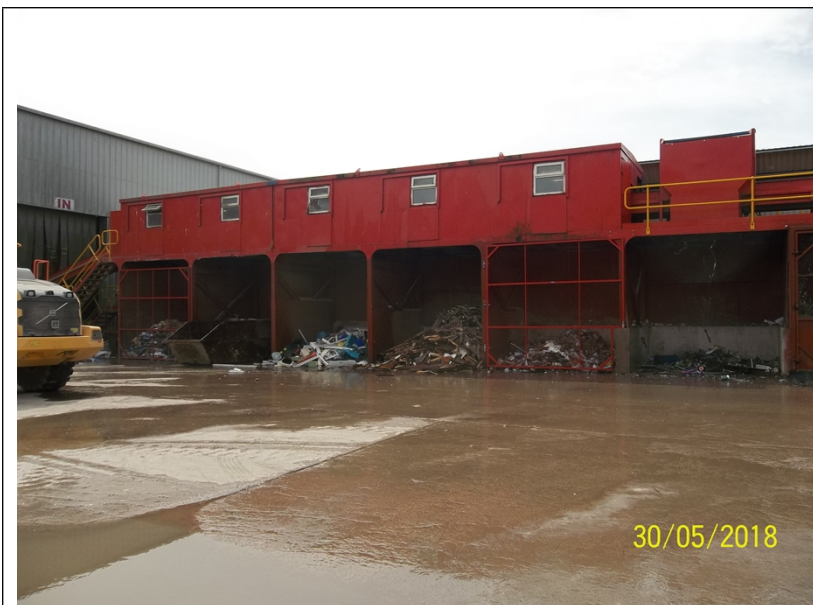
Photo 5: Storage bays beneath picking line.
