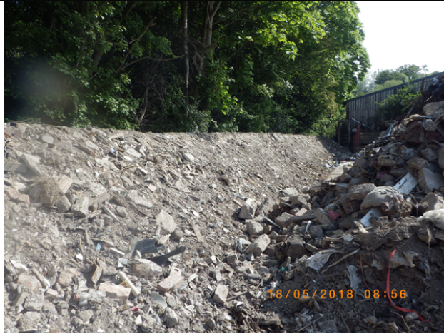
Oversize from the C&D waste (Photo2) and Bund constructed on site (Photo3)
