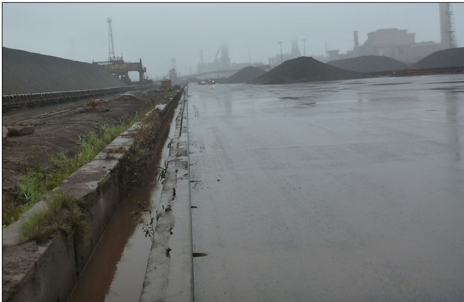
Figure 1. Photograph showing stockyard's surface. Despite heavy rain, the yard's drainage system appears to be functioning correctly with no evidence of significant waste ponding or surcharging drainage systems.
