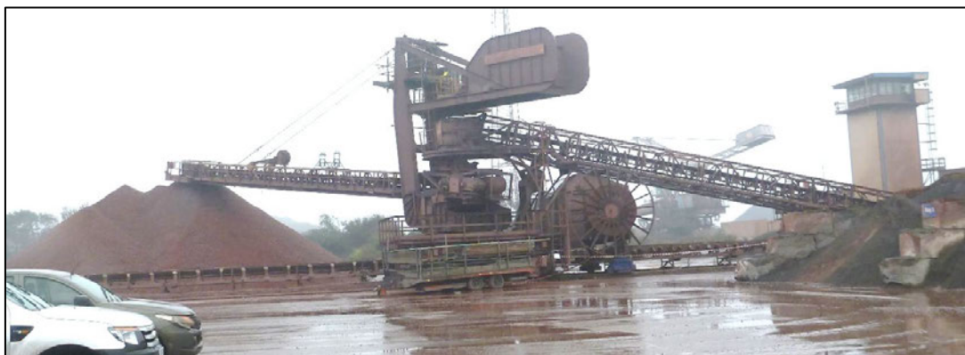
Figure 3. Photograph showing boom stacker.
