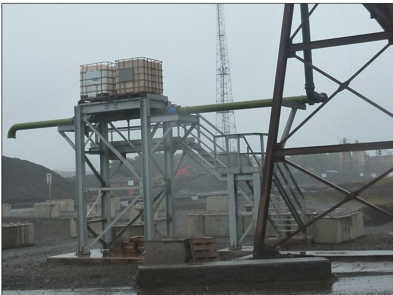
Figure 2. Photograph showing new water filling bowser point within the stockyard's rubble yards, significantly improving the operator's dust management capability.
