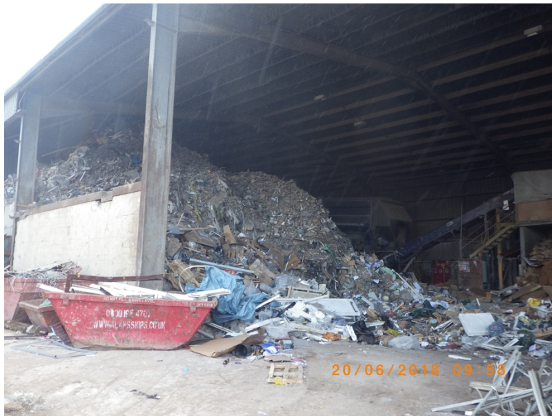
~400T of pre-treated waste in main building
