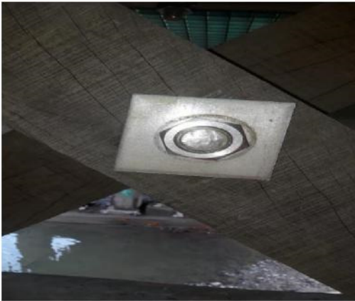
New diagonal restraint timber photo with center bolting installed at Artro. Top of pile 6 T3 replacement works during possession: -
