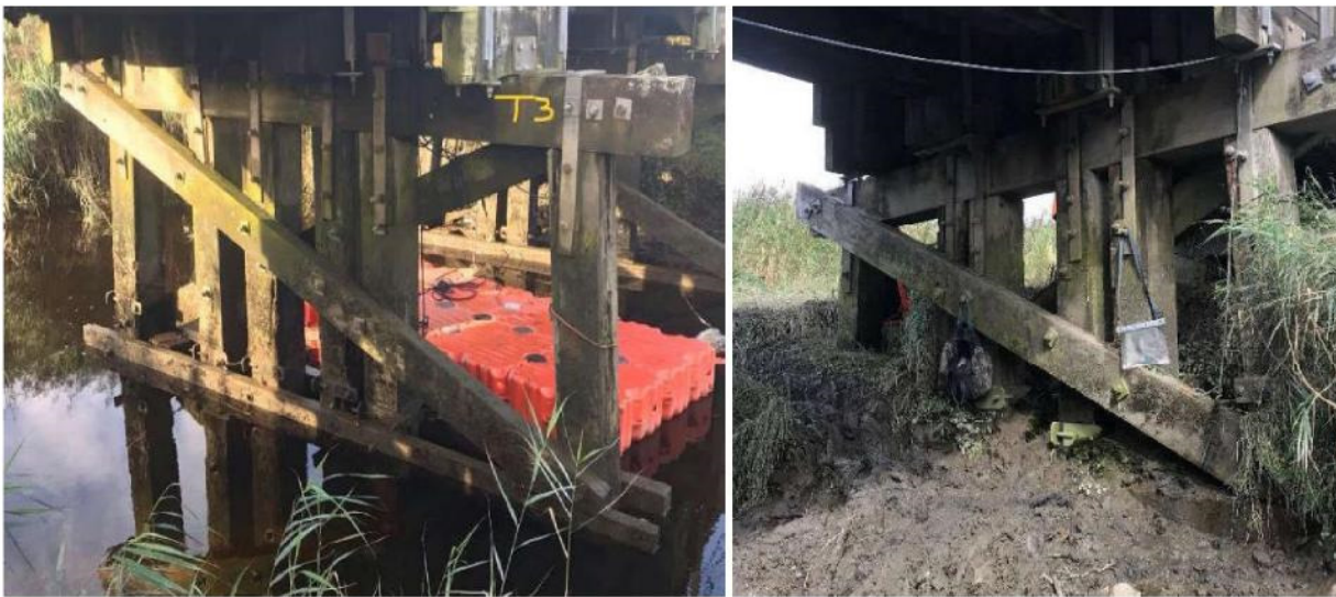
Above picture of T2, T3 showing general arrangement of trestles on this structure.
