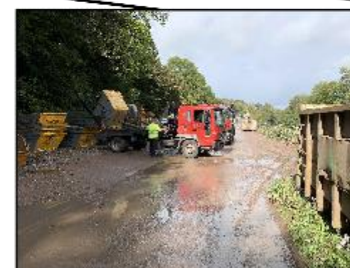
1870 - Empty Skip Storage Area
