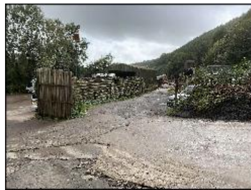
1888 - View South towards Entrance
