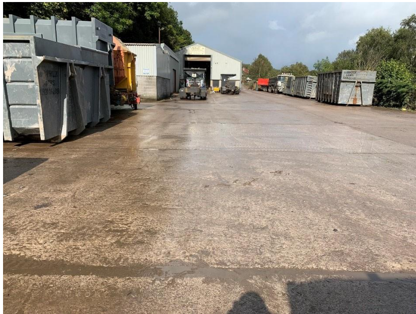
Plate 5-2 Skip storage area in Bottom Yard
