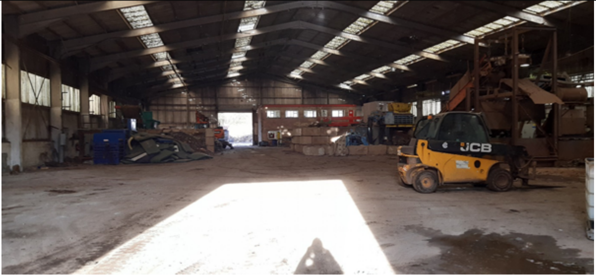
Photo One - Site building
