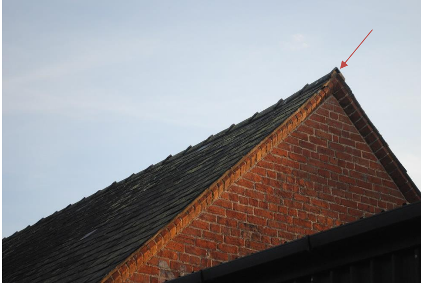
Figure 3: Hole in gable end visible
