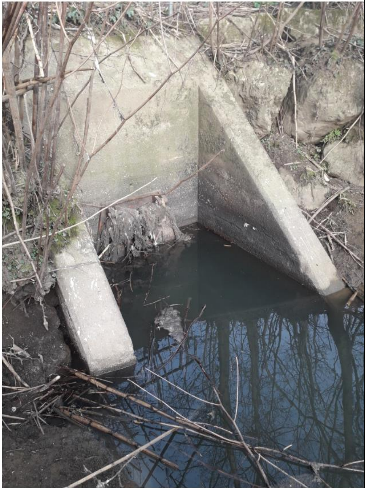
CSO outfall flap valve clogged with debris
