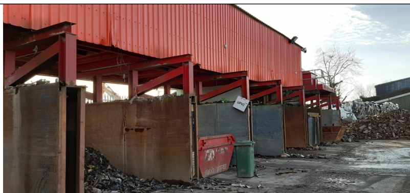
Photo 10 - Separate waste segregation bays at end of waste separation process
