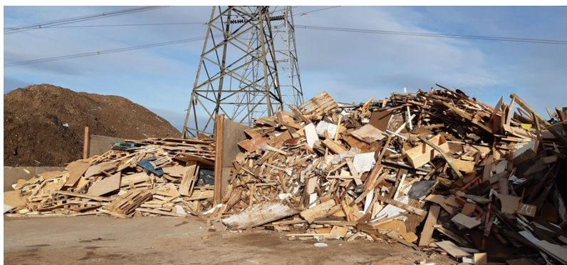
Photo 7 - Stockpile of combustible waste located in close proximity to electrical pylons
