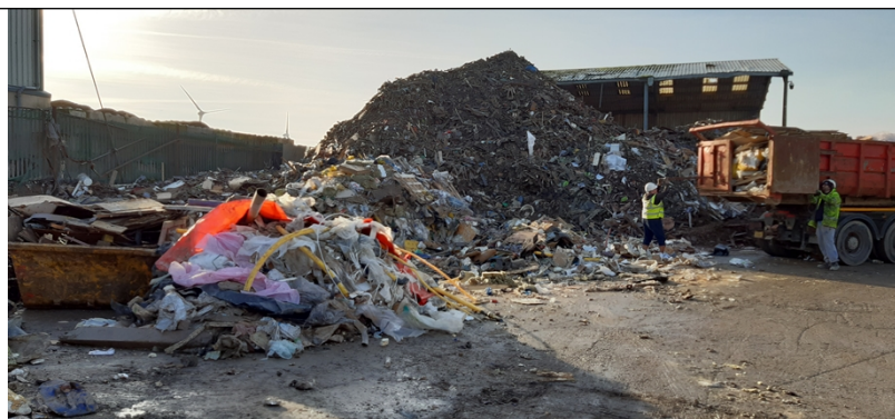
Photo 5 - Stockpile of waste exceeding FPMP guidelines of 4 metres
