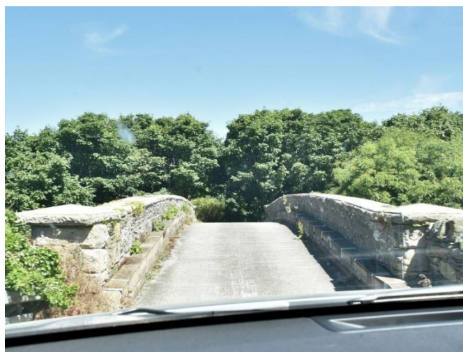
Figure 10 Rail bridge unsuitable for additional cables
