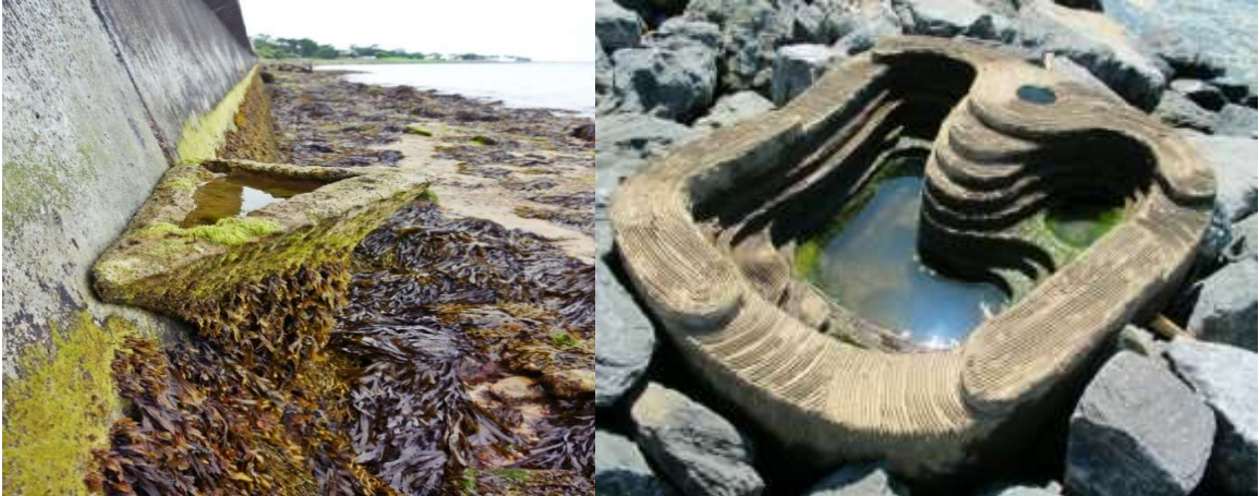
Figure 7.3: (a) 'Vertipools' on a seawall (LEFT) and EConcrete® tide pools amongst rock armouring/riprap (RIGHT).
