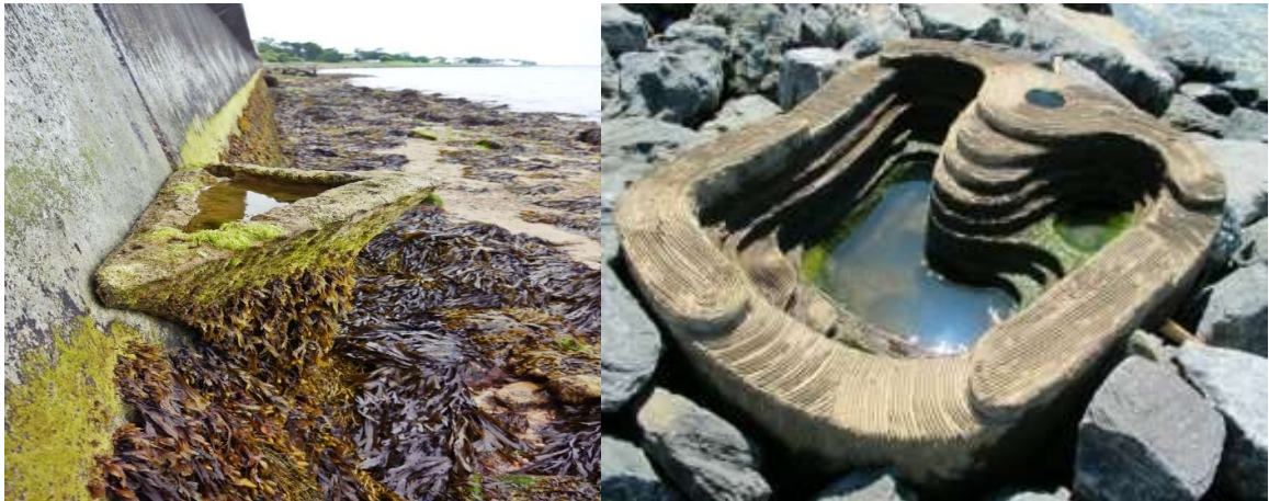
Figure 0.3: (a) 'Vertipools' on a seawall (LEFT) and EConcrete® tide pools amongst rock armouring/riprap (RIGHT).
