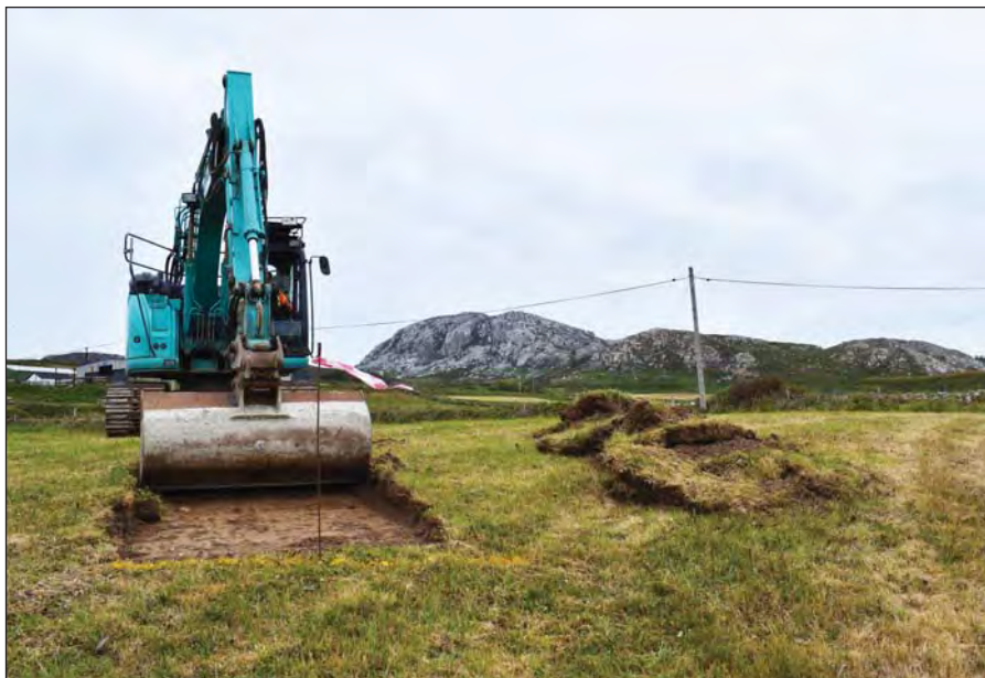
Plate 1. Deturfing with machine (archive reference: G2643_013)
