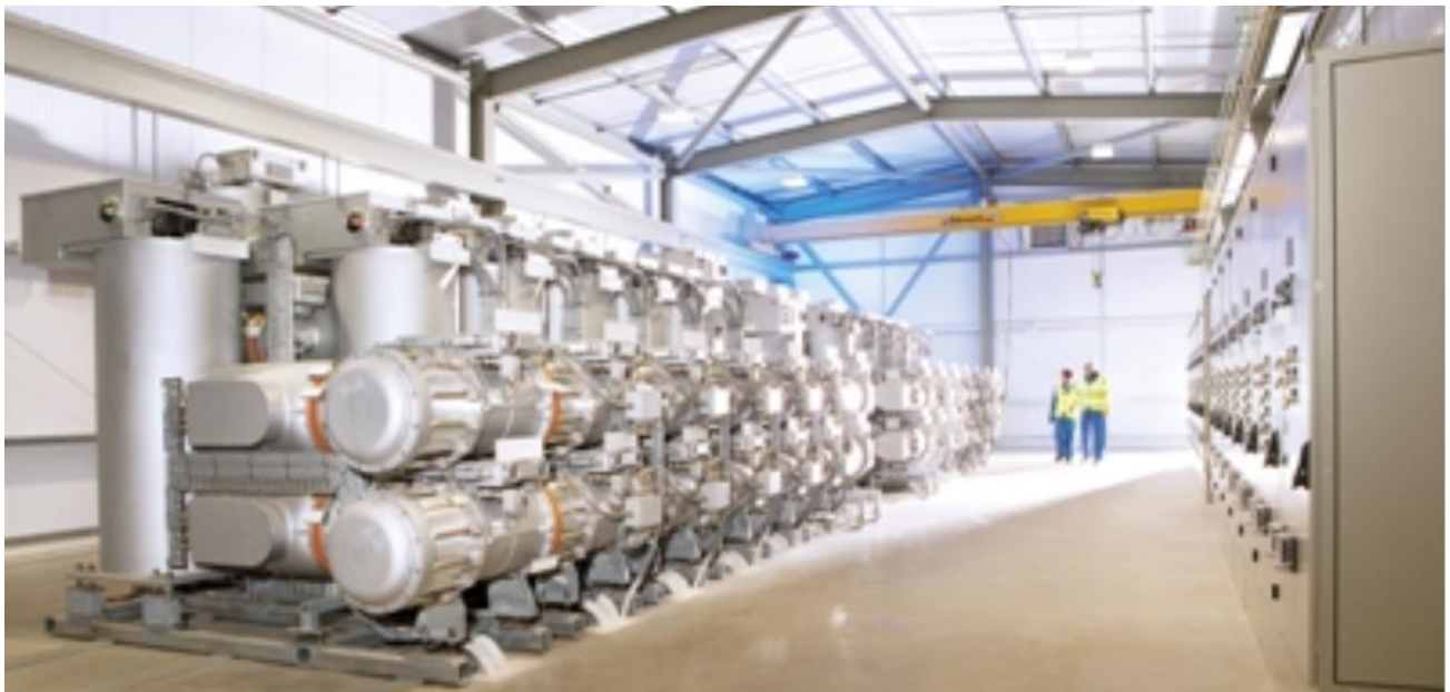
Figure 5 Typical GIS installation
