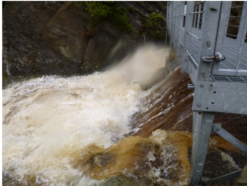
Photograph 1: Point of Abstraction
