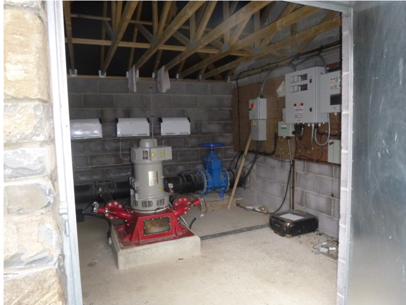
Figure 3: View into the turbine house
