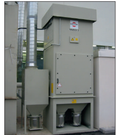
VARIO eco dry separator with exhaust air operation
