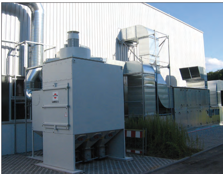
VARIO 5 with spark preseparator and heat recovery system
