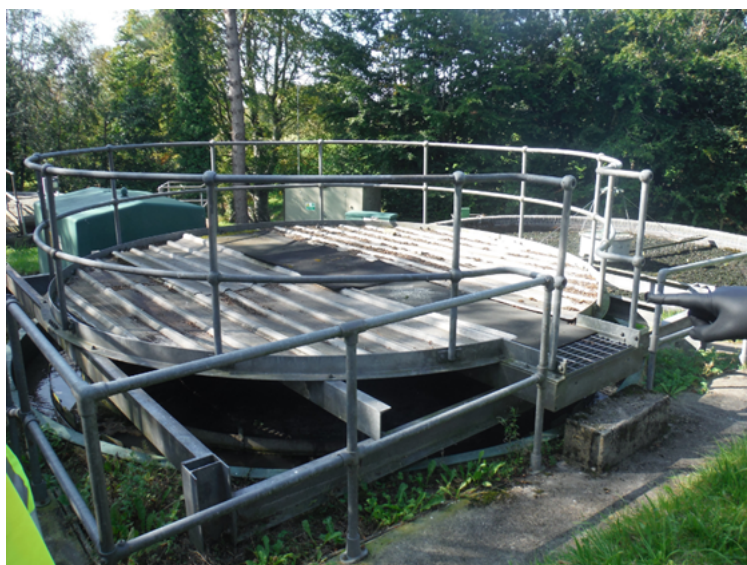
Photo 1: Corrugated sheeting has been used to prevent leaf litter falling into the Primary settlement tank.
