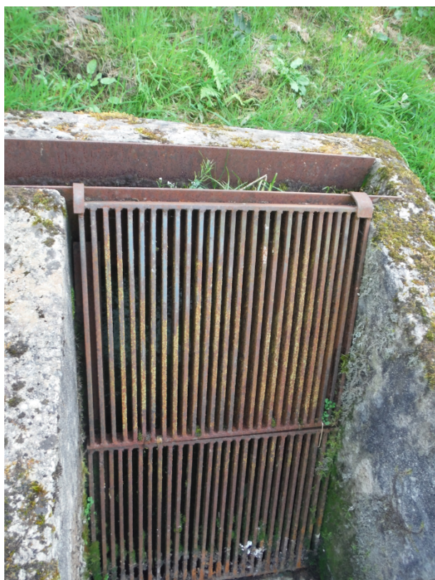
Photo 1: Bar grill at the works inlet. Due to the size of the gaps the grill would appear ineffective in being able to capture small pieces of rag and debris.
