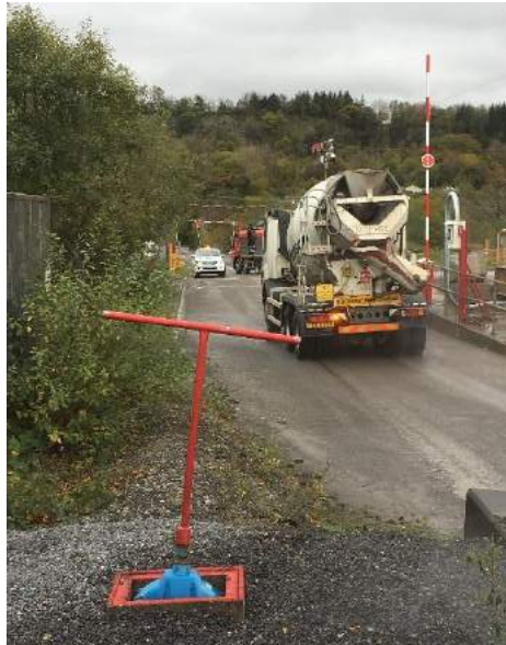
Figure 2.2 Photograph of stopcock used to manually divert water for use in dust suppression and wheel washing
