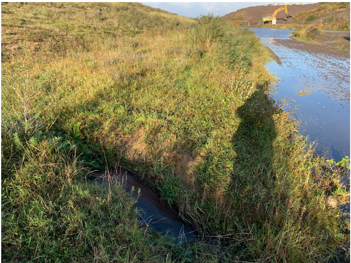
Plate 6-1 Surface water ponding between toe of MCL (left) and Biocell (on right). Partly being caused by drainage channel overtopping at toe of MCL in foreground.
