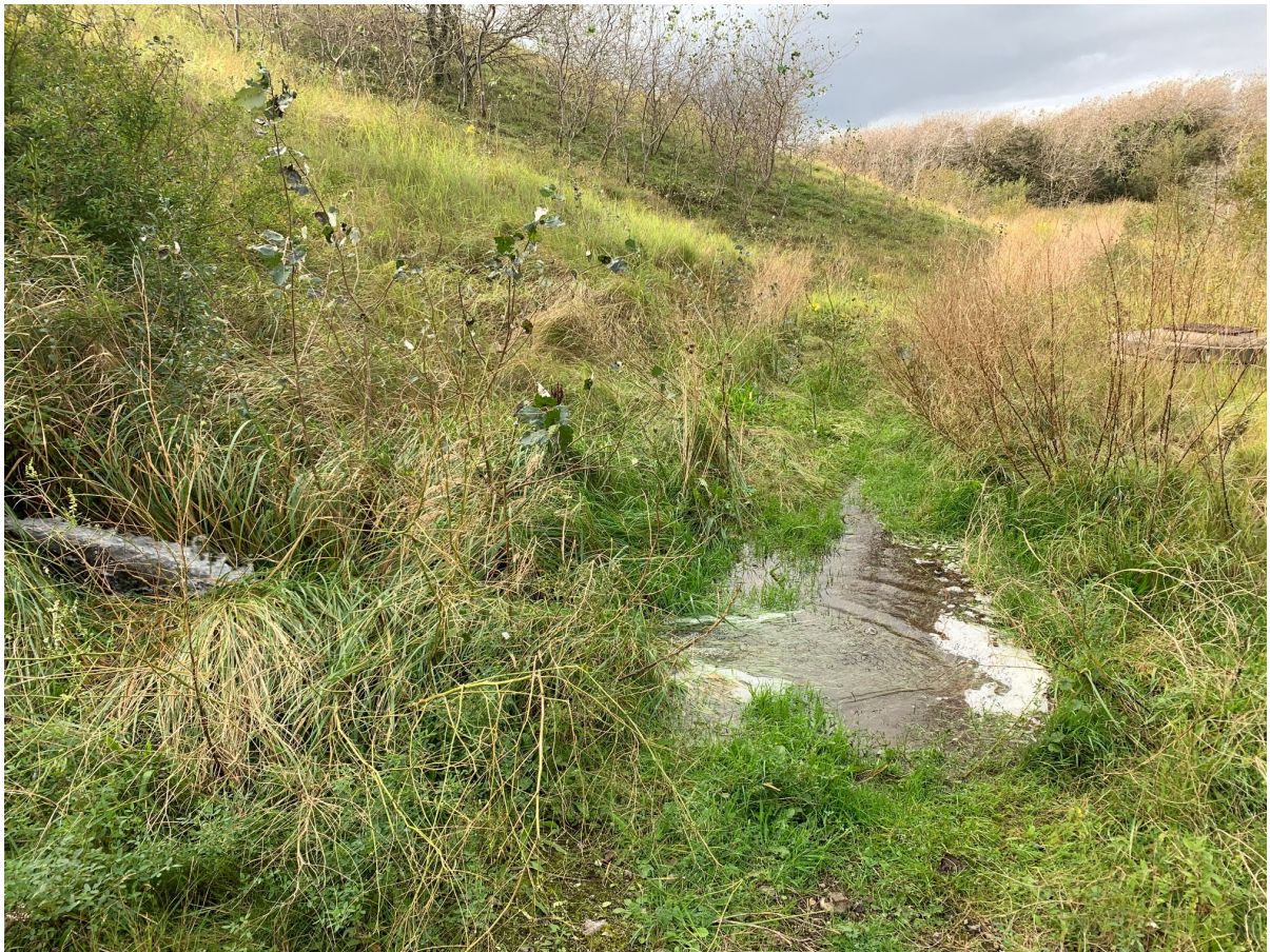
Plate 6-2 Emission from Pond 2 (left) at toe of MCL draining northwards towards P10/P11 (Note recharge chamber on right of photo)
