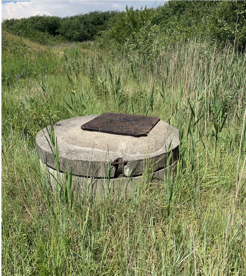
Plate 4-4 One of the two recharge chambers at toe of MCL
