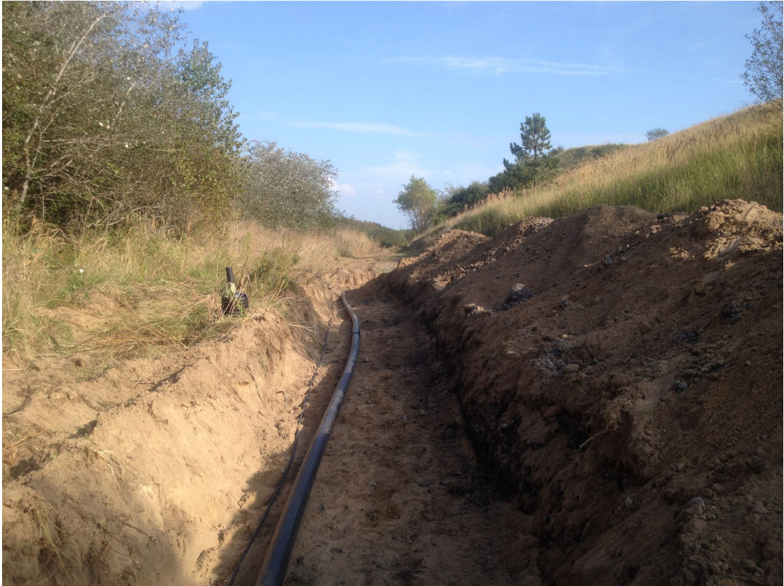
Plate 4-2 Pipework in trench along toe of MCL
